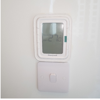
Electrical Switches and Power Points
